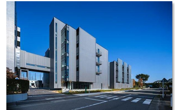
Parker Innovation Center (Opening in April 2025)
